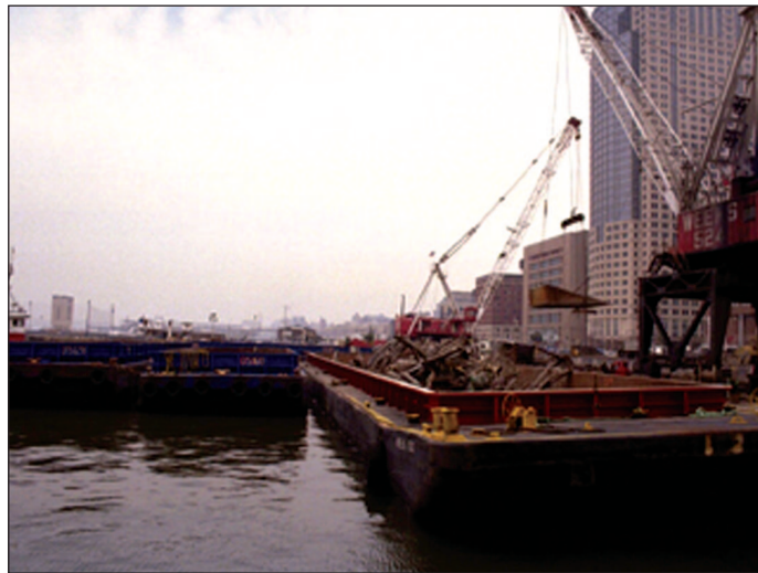
Source: FEMA Photo Library.
