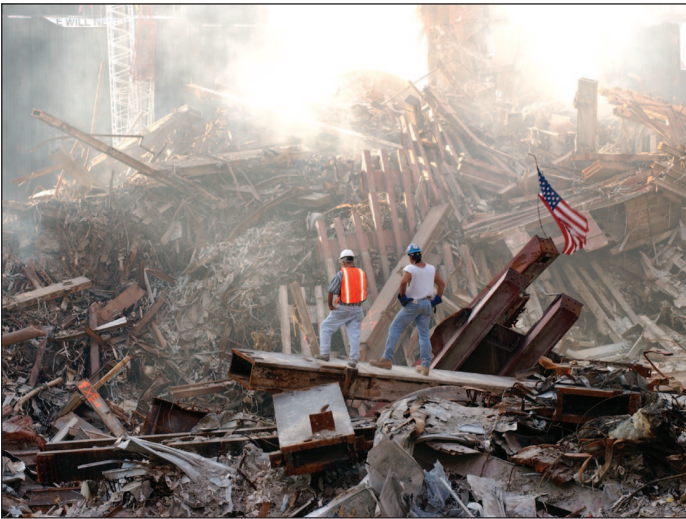
Source: FEMA Photo Library.
