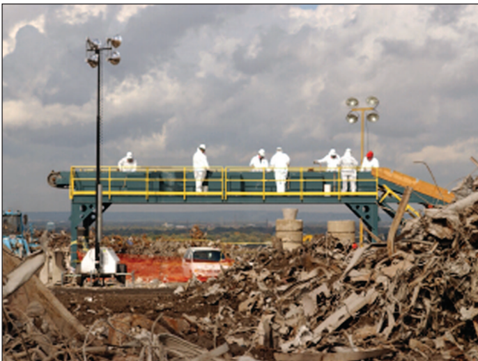
Figure 4: Debris Screening and Inspection Operations
