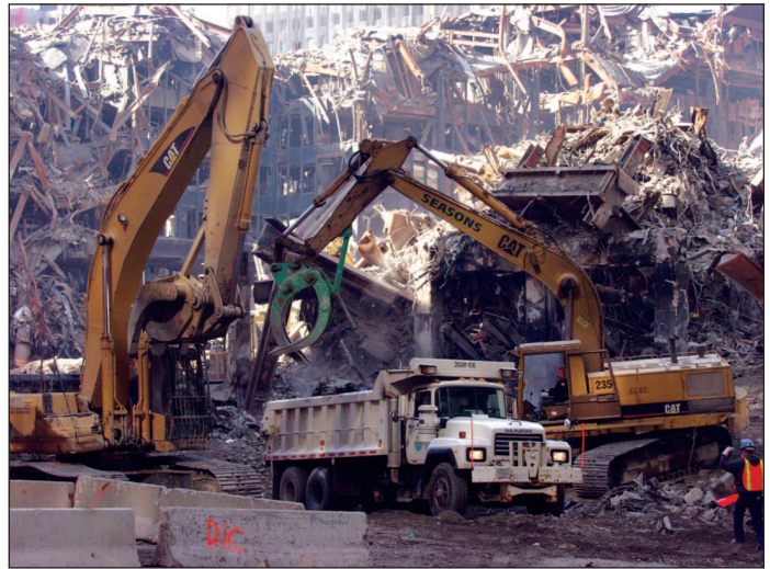
Source: FEMA Photo Library.
